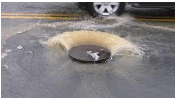
Overflowing sewer manhole during wet weather
