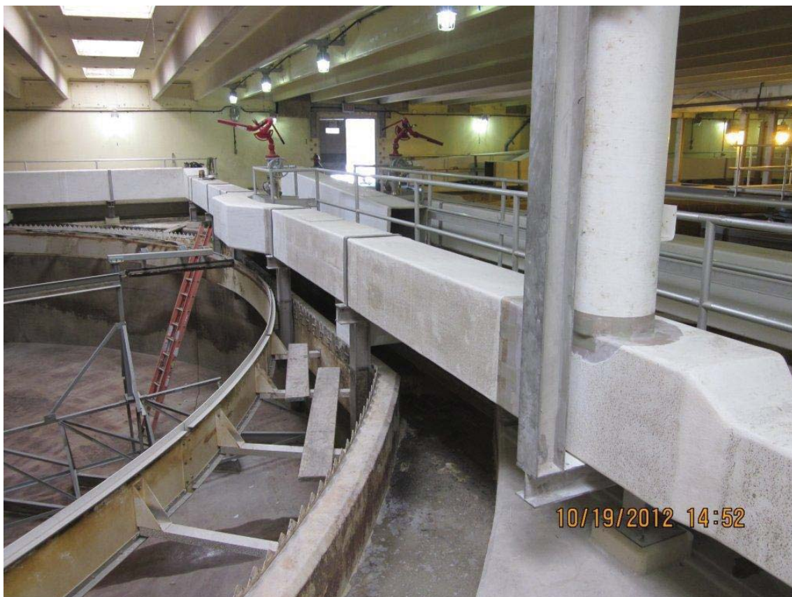
Installation of Clarifier Perimeter Fiberglass Duct
