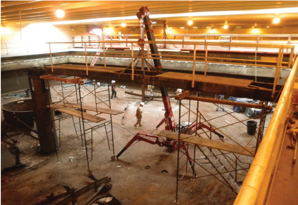
Mechanical Demolition of Clarifier No. 4
