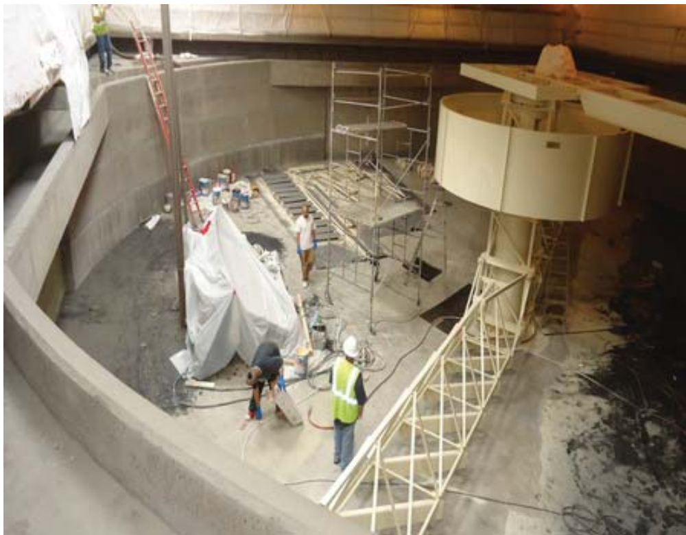
Coating of Steel Components of Clarifier 2
