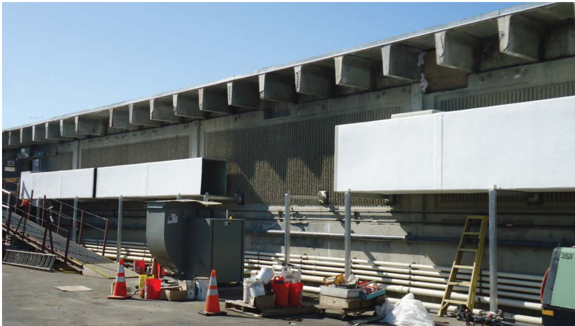
Exterior Duct Erection
