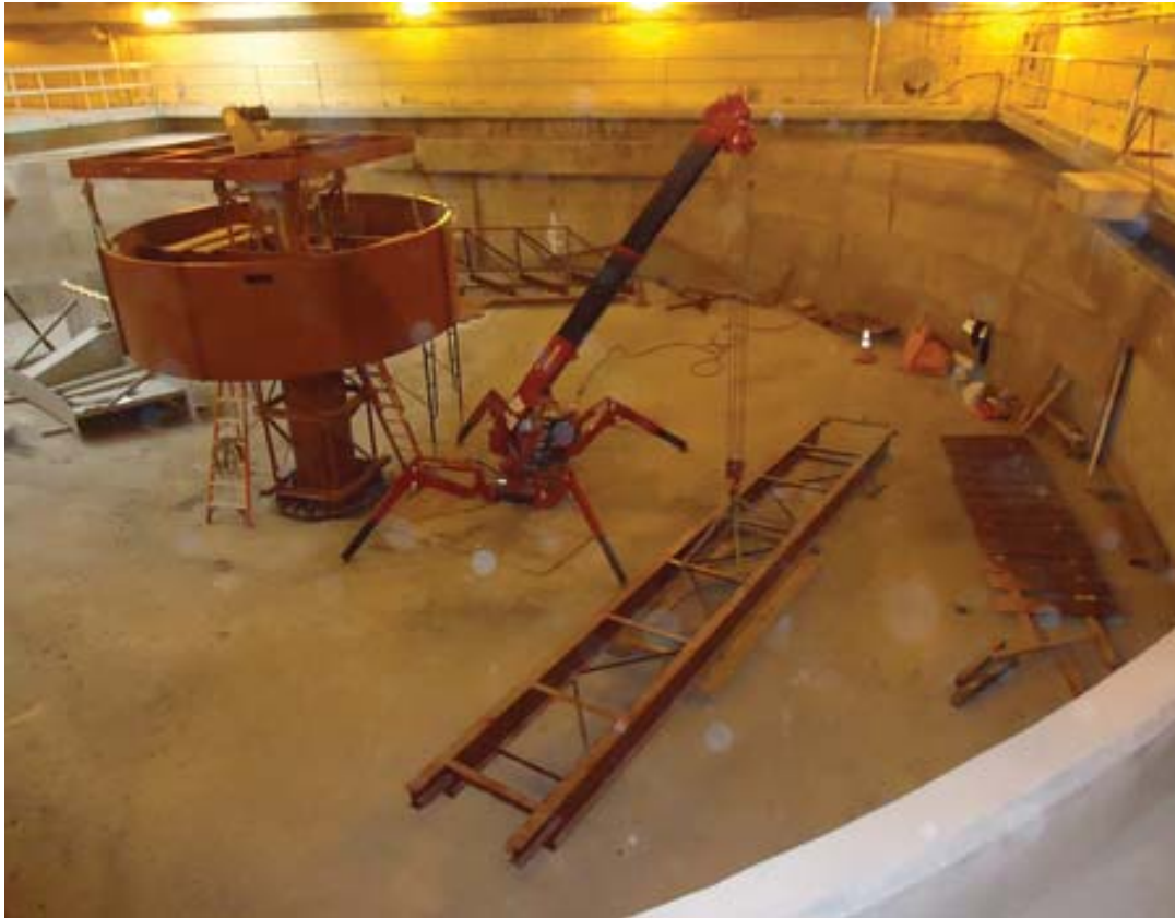
Mechanical Erection of Clarifier 2
