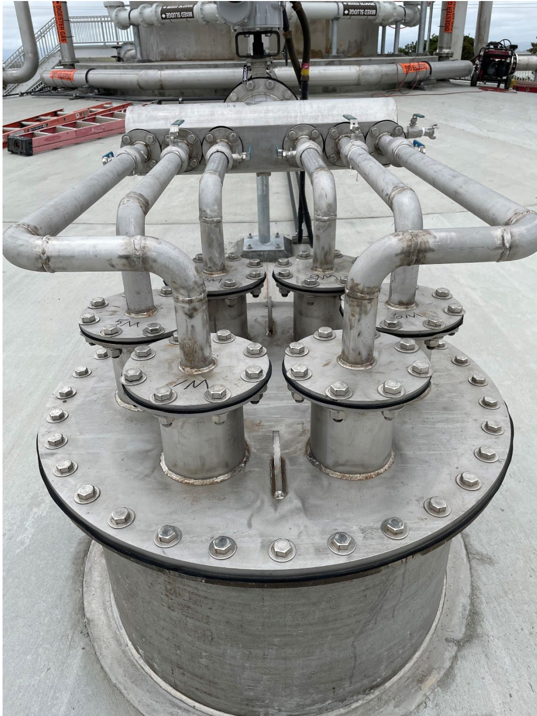
Gas Lance Mixing Header – Digester 7
