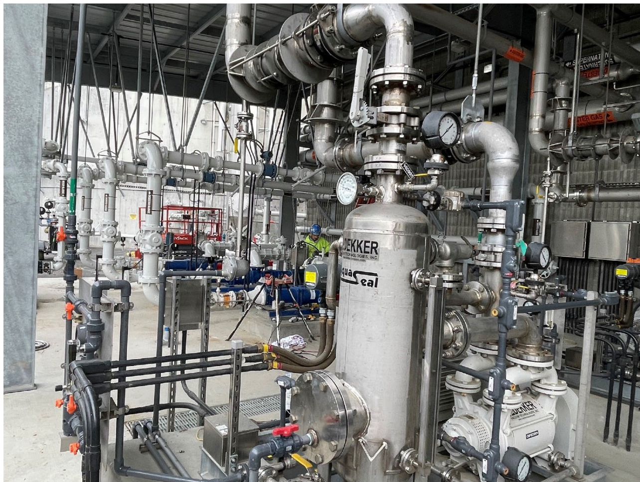
Pumps and Piping for Digester 7
