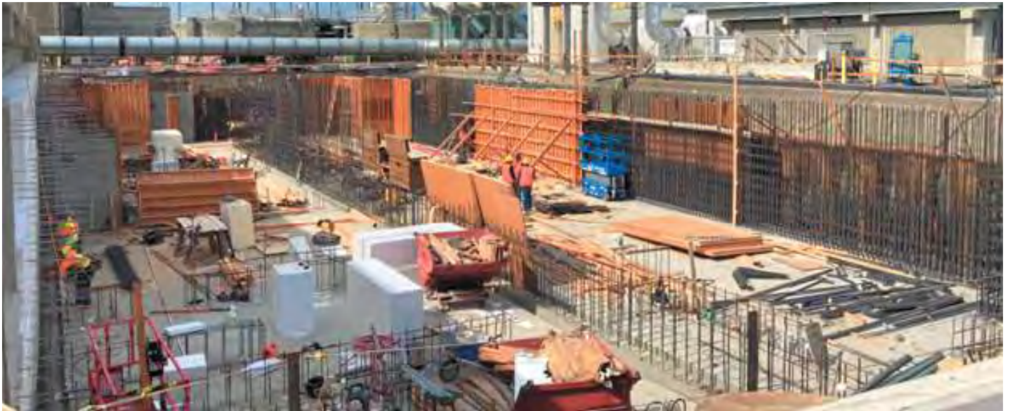
ETSU Phase 1A - Aeration Basin Modification Project, New Aeration Basin 8
