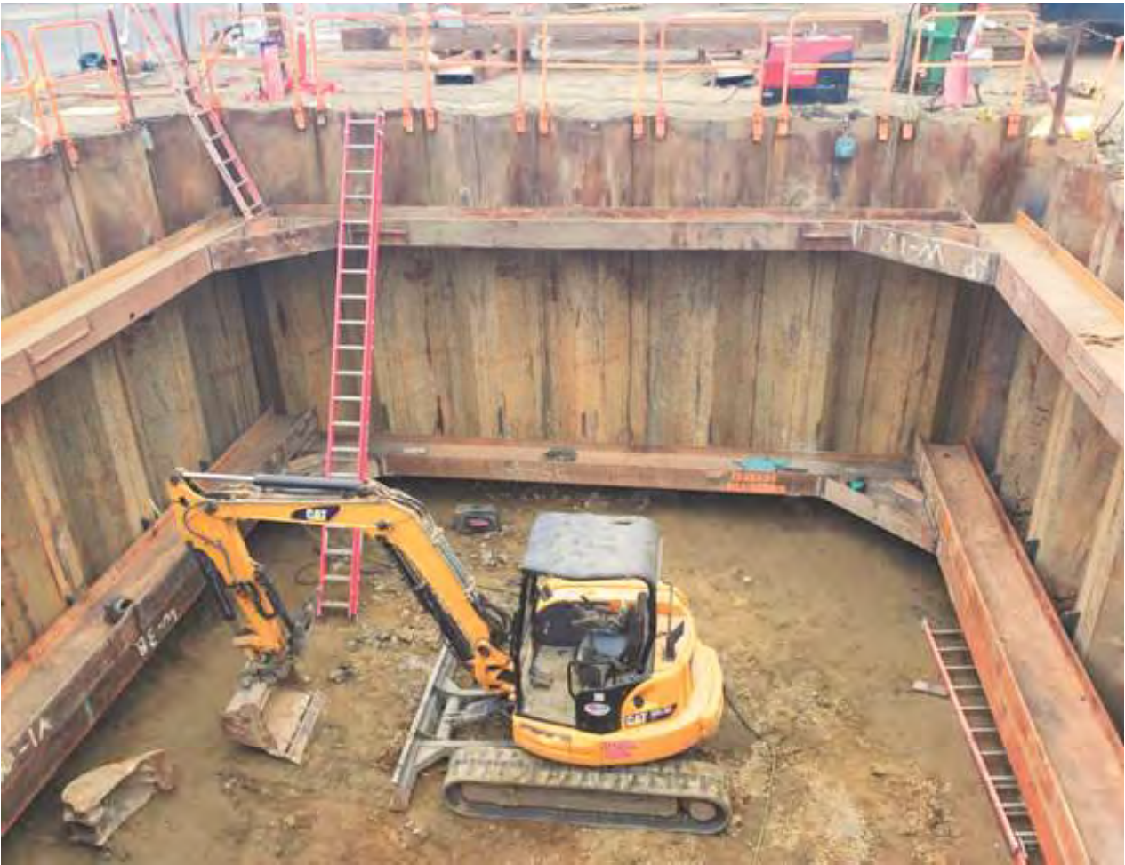
ETSU Phase 1A - New Pump Station
