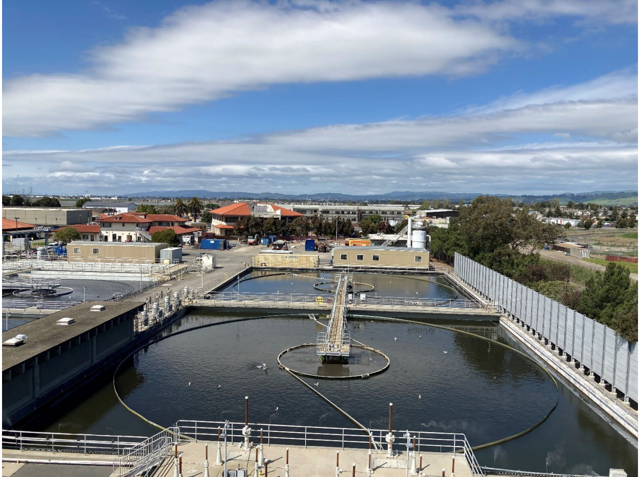
View Northward over the Secondary Clarifiers
