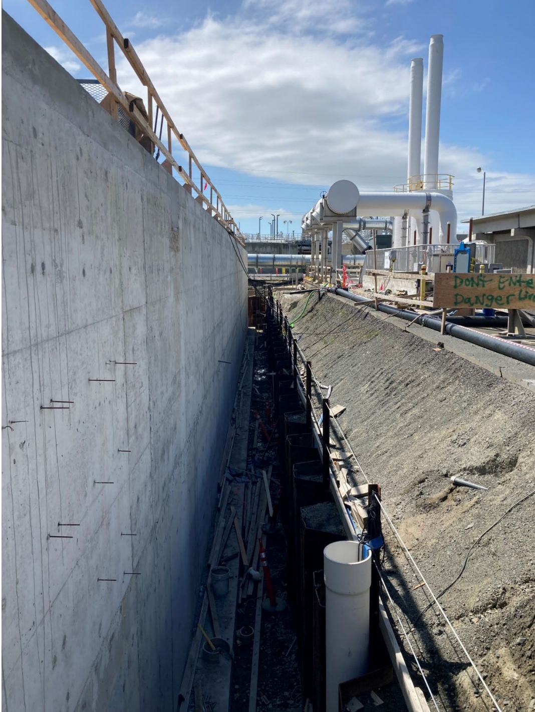
ETSU Aeration Basin Project
