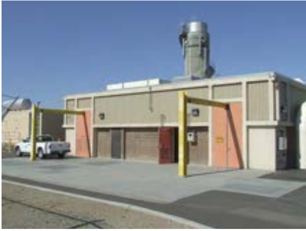
Irvington Pump Station
