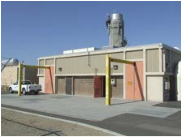
Irvington Pump Station
