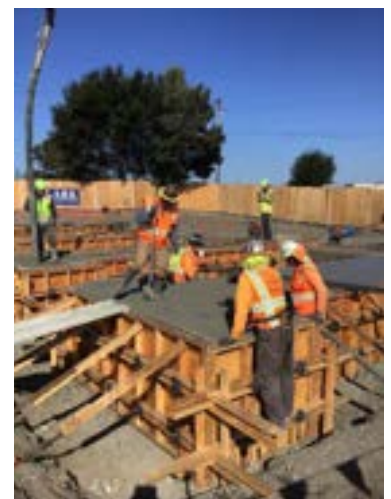
Standby Power Project Construction
