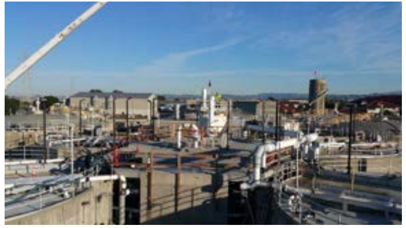
Digester maintenance and rehabilitation
