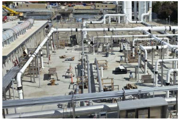
Plant Project: Aeration Basin Construction
