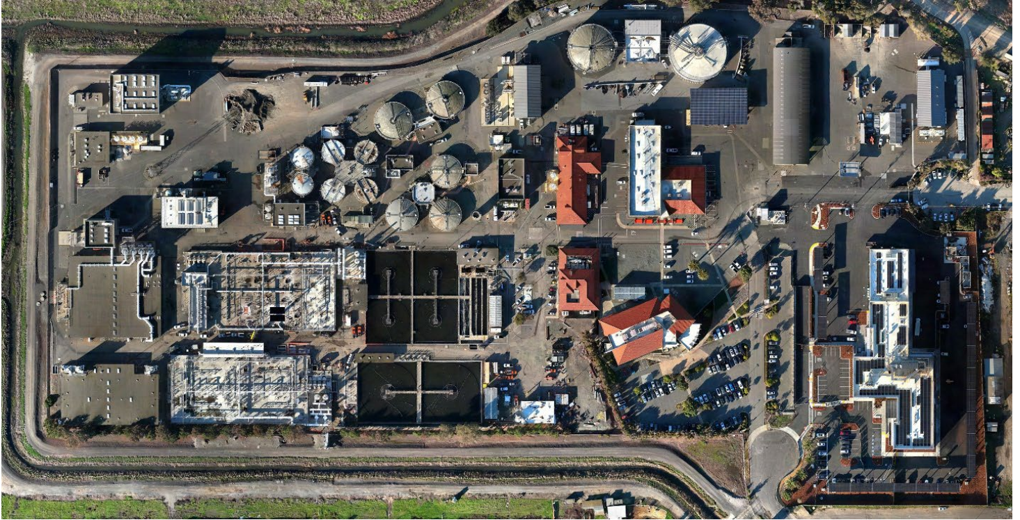
Aerial View of the Treatment Plant
