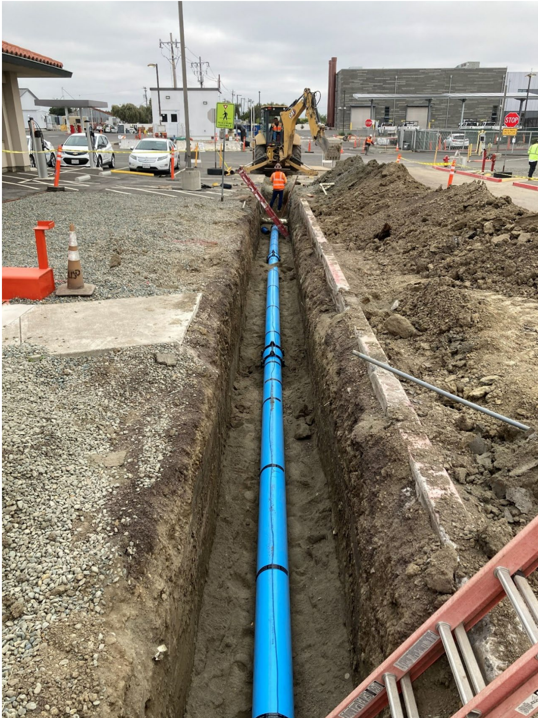
Installation of New Water Line to the Collection Services Building
