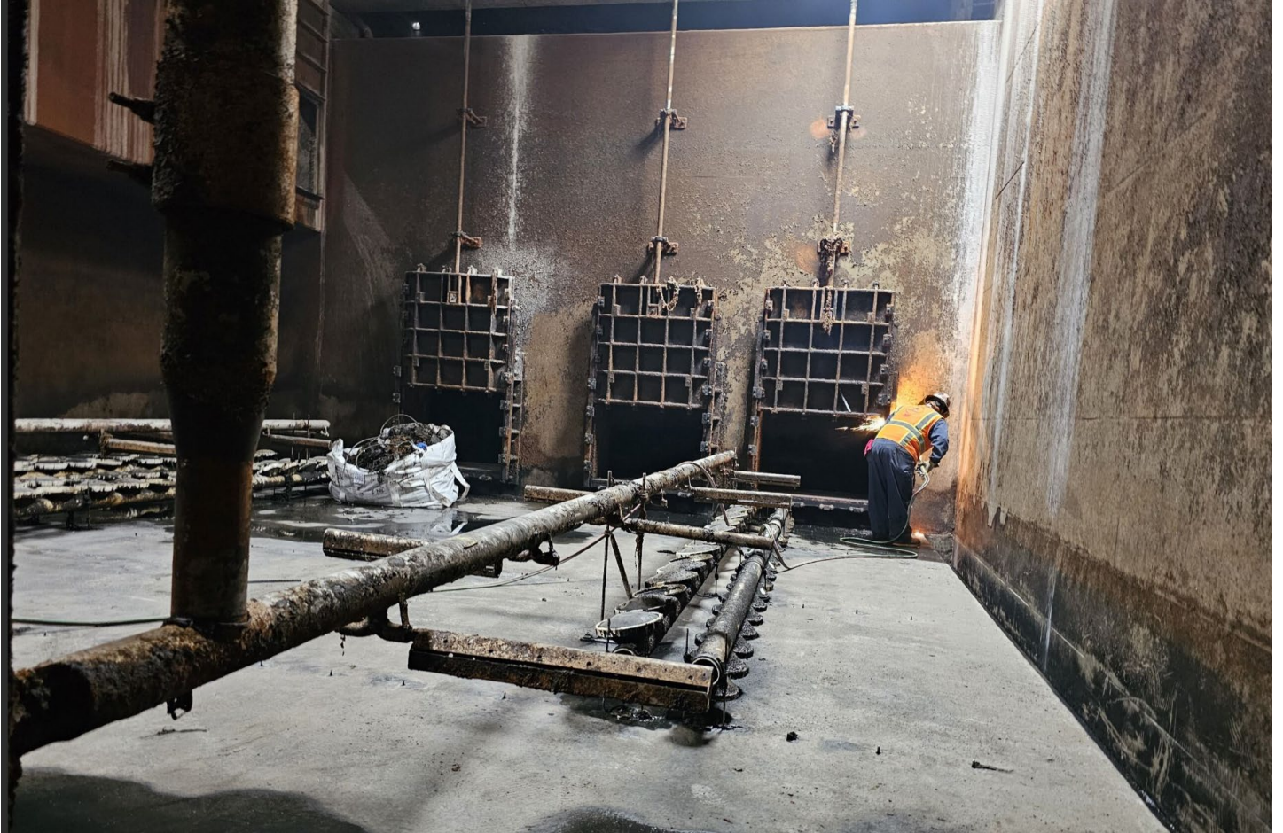
Westerly Aeration Basins Under Construction
