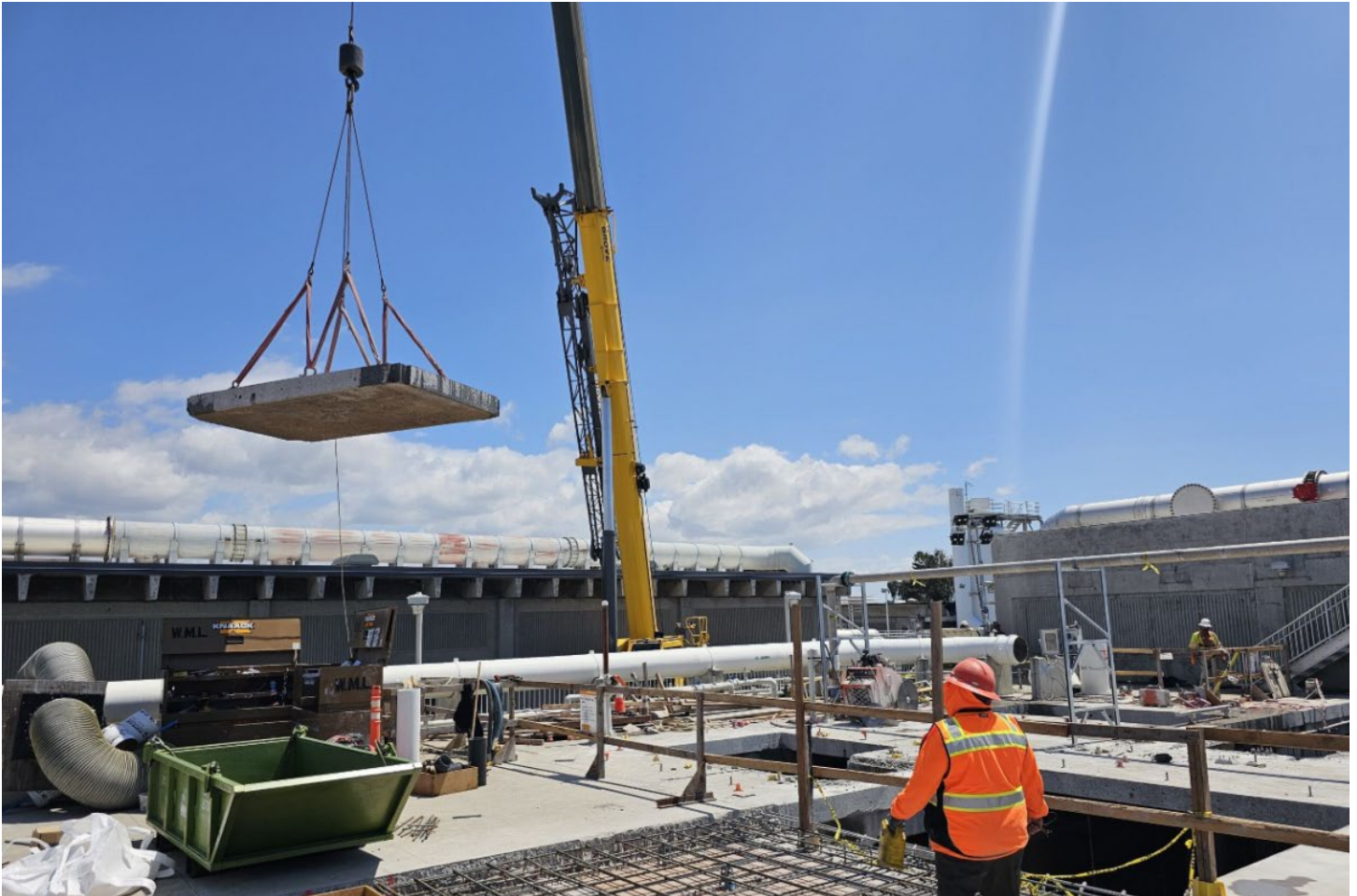
Construction of New and Refurbished Aeration Basins
