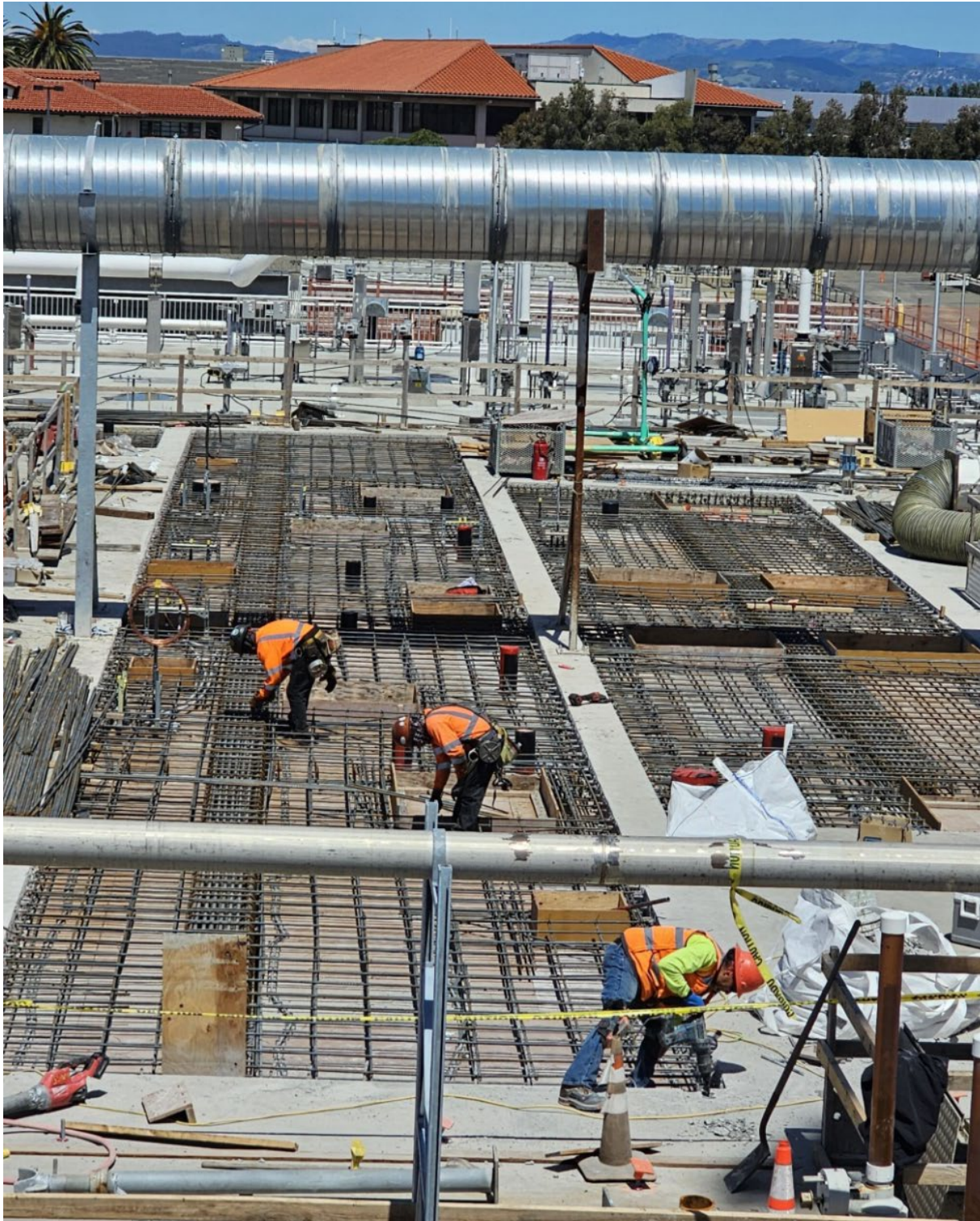
Westerly Aeration Basins Under Construction
